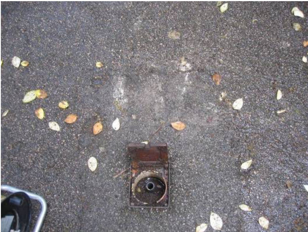
Plate 44 Scarborough South Cliff H5
