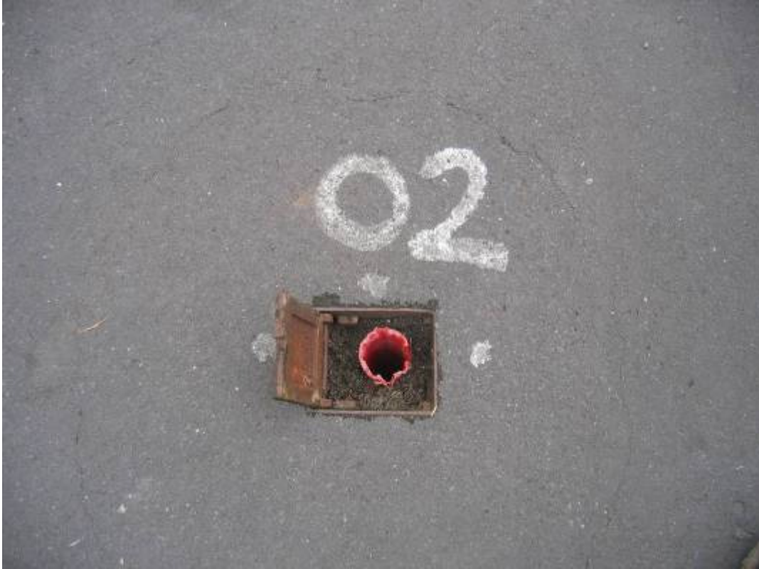
Plate 29 Scarborough South Cliff H4 (AA02)
