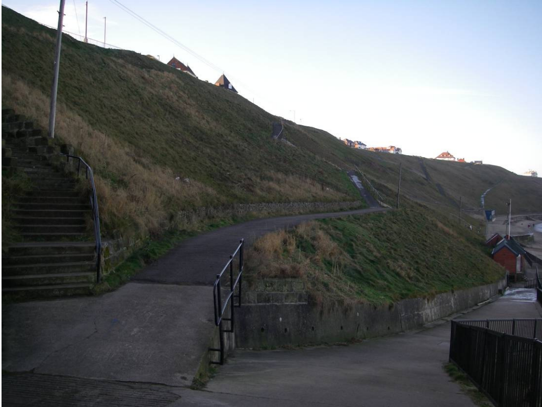
Plate 7 Site view of West Cliff slopes looking west.
