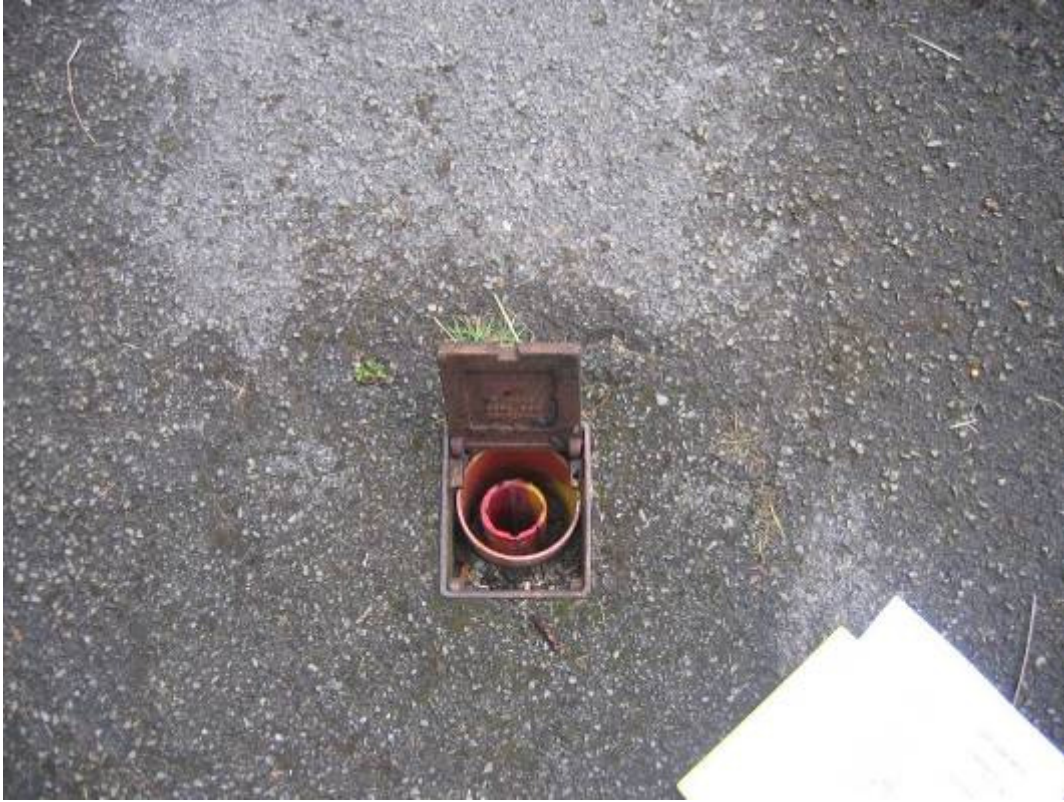
Plate 37 Scarborough South Cliff D3 (AA08)
