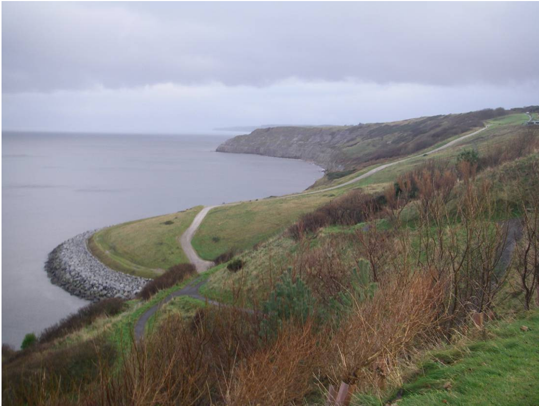
Plate 21 Site view looking south towards Holbeck Gardens and Holbeck Cliff.
