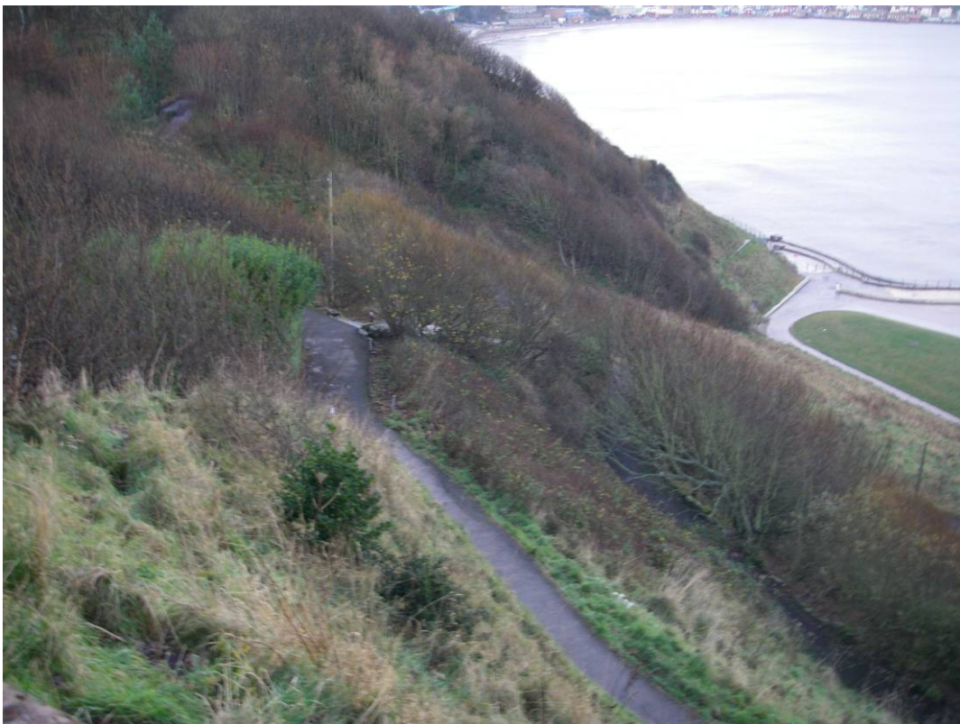
Plate 22 Site view showing steep slope angles above South Bay Pool Cliff.
