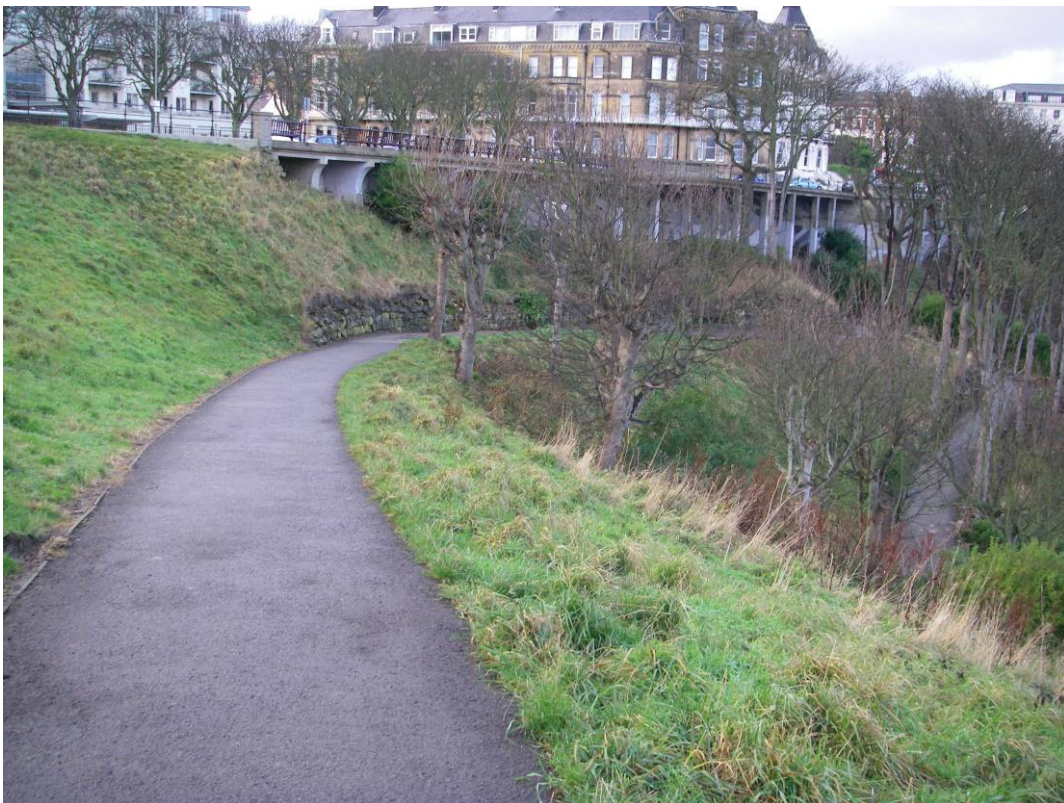
Plate 24 Site view looking north at arcuate embayment at South Cliff Gardens.
