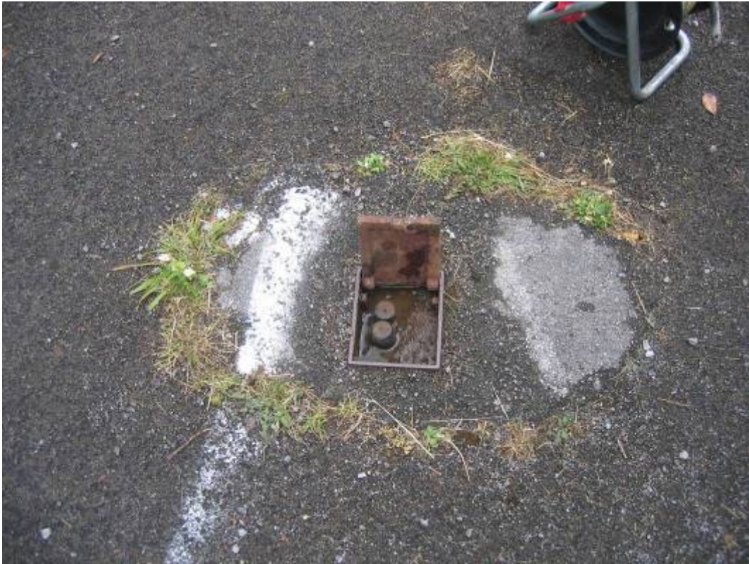
Plate 59 Scarborough South Cliff Bh1
