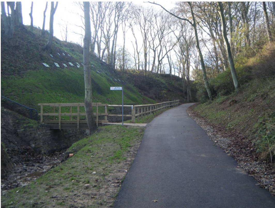
Plate 35 Site view looking up Martin's Ravine. (Remediated slopes on left).
